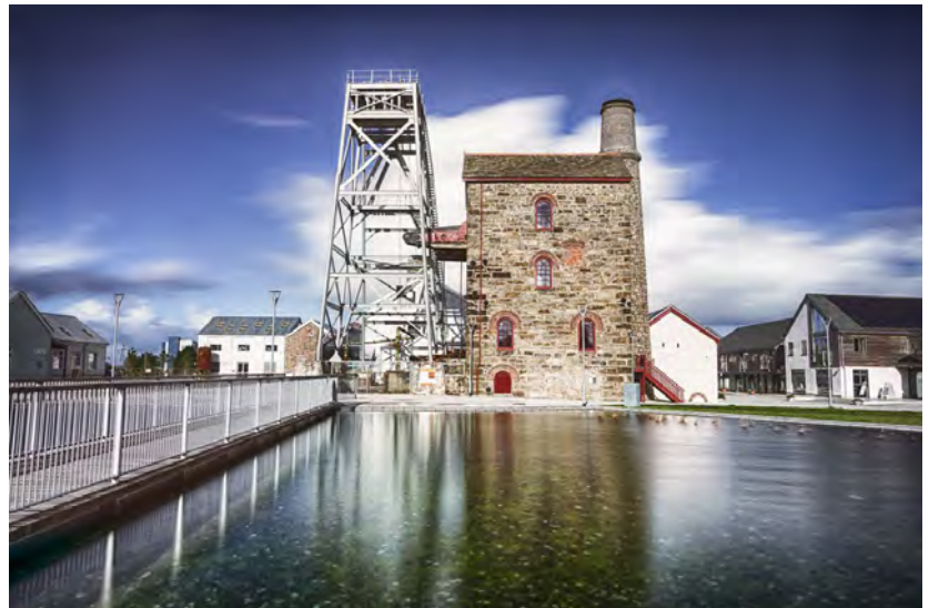
Photo 5: Robinsons Shaft at Heartlands.
