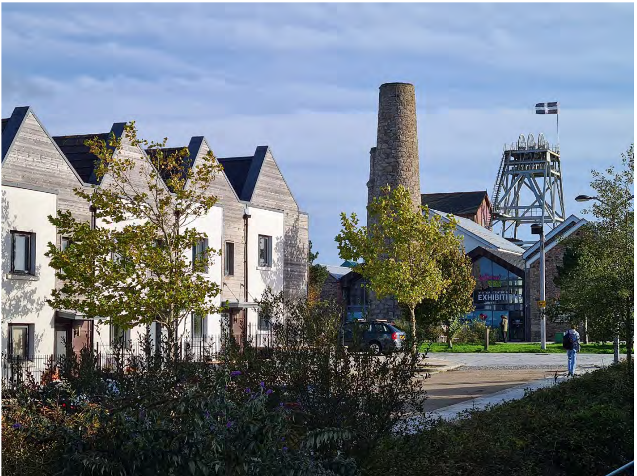
Photo 7: Robinsons Avenue looking towards Robinsons Shaft and Engine House, showing how important views of tall heritage features contribute to the local sense of place.
