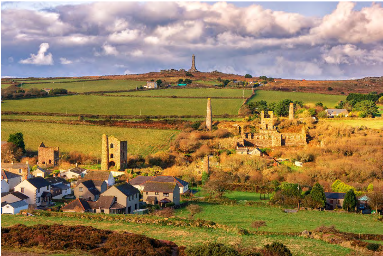
Photo 6: Carnkie, looking from West Basset Mine northwards towards West Basset Stamps and the Basset Monument, over the Great Flat Lode.
