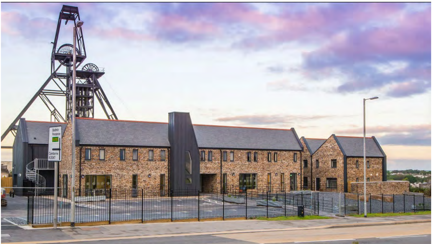
Photo 8: Chi Winder and Chi Vesta crisis accommodation on Dudnace Road, Pool. Winner of Building Forum for Devon and Cornwall Building of the Year Award 2019. Functionally excellent with a design that is sensitive to its distinctive location.
