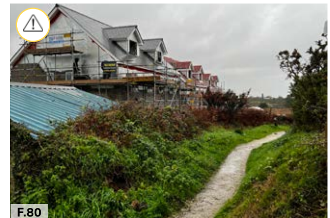
Figure 80: Recent development that is insensitively sited on an exposed site in rural Carn Brea and does not adhere to the local vernacular styles of Carn Brea.
