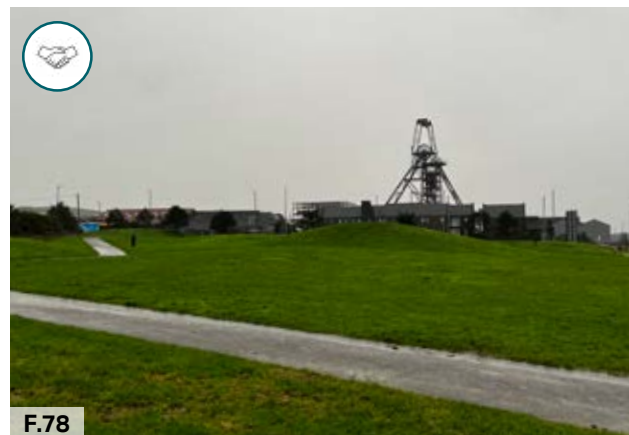
Figure 78: New mixed use development on the Dudnace Lane allocated site is anticipated to bring further employment opportunities and revitalisation for this part of Pool.
