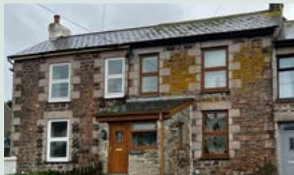
Front extension with adequately proportioned, pitch of roof matches the original property
