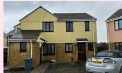
Extension overly dominates the front elevation of the property
