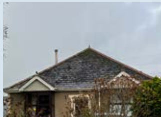
Grey slate hipped roof with red clay ridges and gabled dormers
