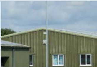
Corrugated iron pitched roof
