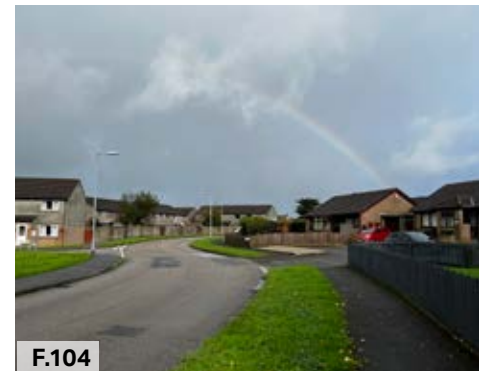
Figure 104: Building lines are consistent but follow gently meandering roads and cul-de-sacs, with subtle variations in building setbacks and orientation, Treloweth Way.
