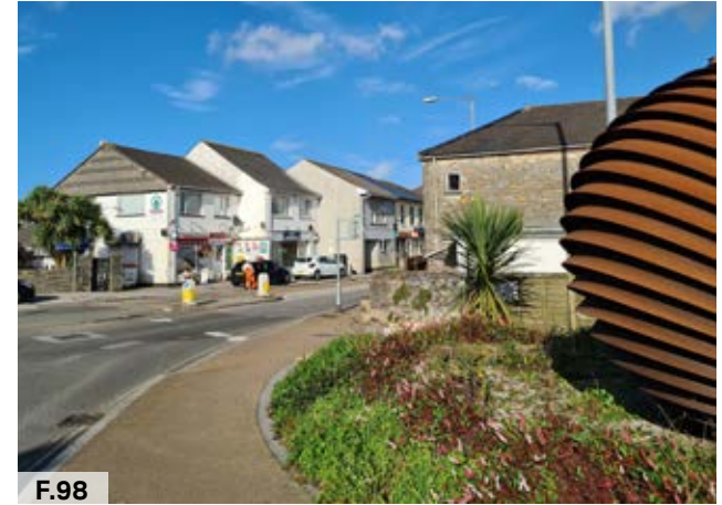
F.98 Figure 98: Landscaping and large tin sculpture marks the gateway into the heart of Pool village at the intersection of Station Road and Fore Street, whilst honouring Pool's tin mining legacy (Source: Carn Brea NDPDG)
