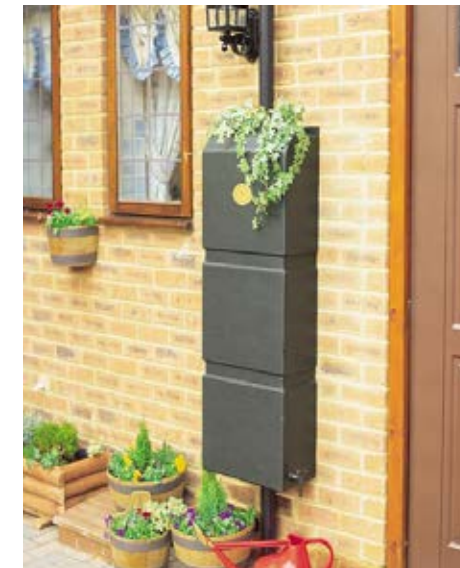
F.133 Figure 133: Example of a gravity fed rainwater system for flushing a downstairs toilet or for irrigation.
