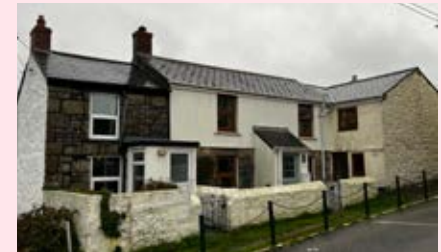
Front porch extensions are out of scale and dominate the front elevation of properties
