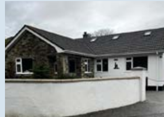
Cross-gabled grey slate roof
