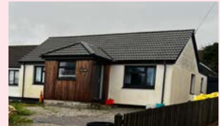
Unsympathetic use of timber on extension that is out of character
