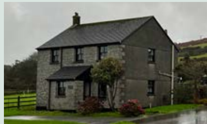
Sympathetic use of material on extension that matches the primary frontage
