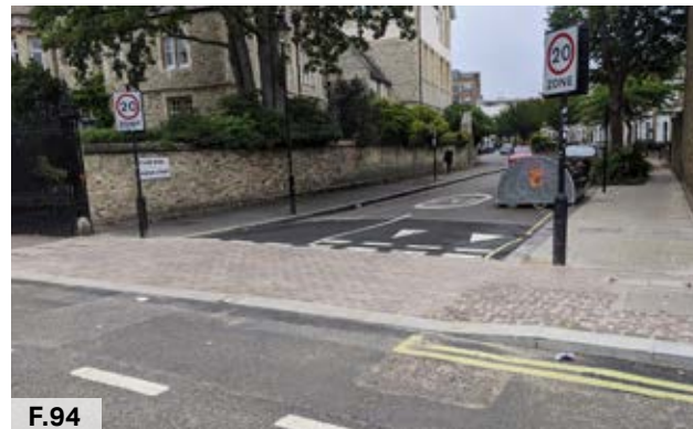
Figure 94: Example of a raised junction at the entrance to a residential street as a way to slow traffic entering onto a residential street.
