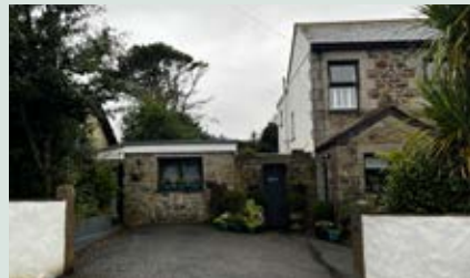
Garage conversion with material that is in-keeping with the main property
