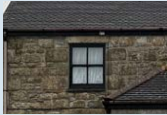
Timber sash window
