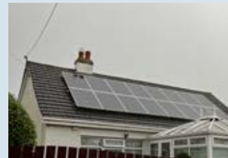
Grey slate roof with solar panels
