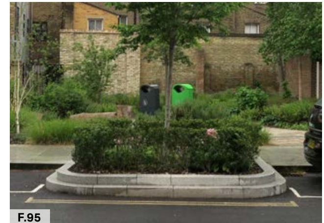
Figure 95: Kerb build out with street greening and SuDS installation, double kerb to prevent vehicle overrun.
