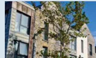
Local stone with white render, timber boards and iron panelling
