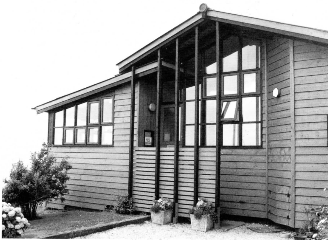
Single storey dwelling at Portwrinkle
