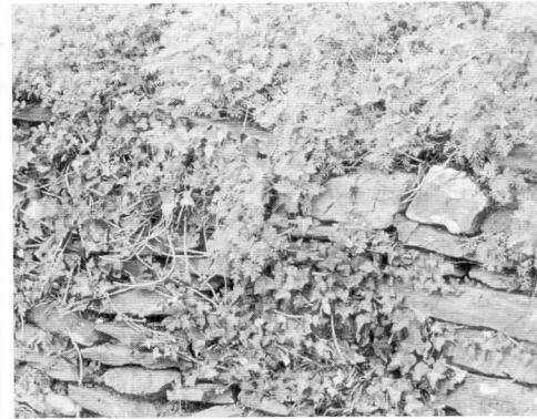
Retain existing site features whenever possible. Match local laying patterns if constructing new walls.
