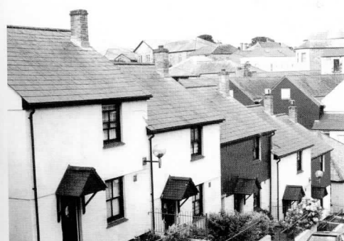
A terrace of simple modern cottages in Liskeard, stepping down a steep gradient in the traditional manner.
