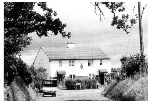
A good example of low cost modern housing at Lerryn.
