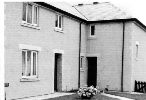
Note the use of simple ashlar lintels and quoins in conjunction with a warm coloured pebbledash.
