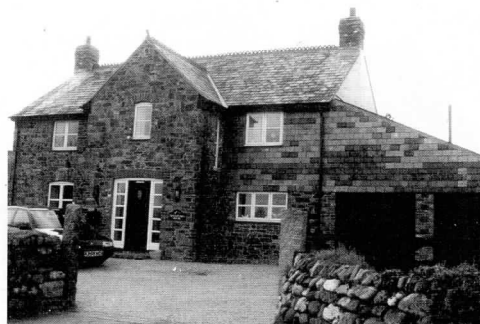
A large detached family house built of local stone with slate hanging.
