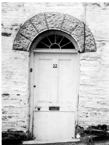
Retain and repair original joinery. Note the fan light is positioned over the door, and the correctly detailed glazing pattern. Repairing this door would be cost-effective in comparison to replacing it with a new one.
