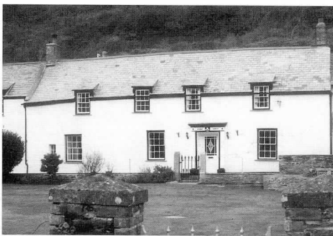
The use of dormers can reduce the apparent scale of a building to one and a half storeys.
