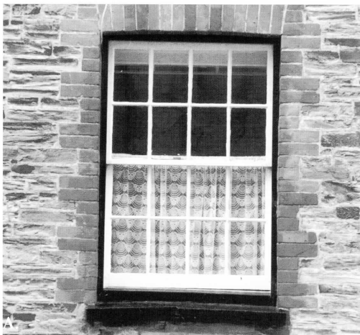
A. Georgian 16 pane vertical sliding sash window.
