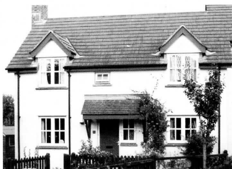
Modern cottage style house. The barge boards are rather too deep, but the overall effect successful.
