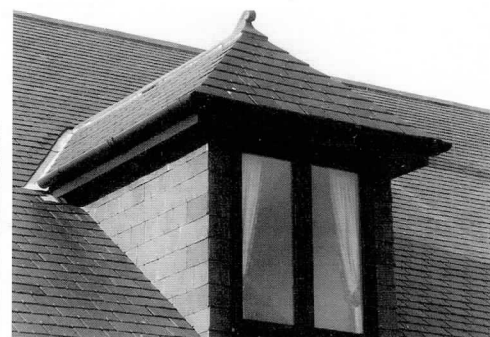
A modern hipped dormer with mitred real slate hips and cheeks. The fascias are rather too deep on this example. The use of hipped dormers helps to merge the element into the roof.
