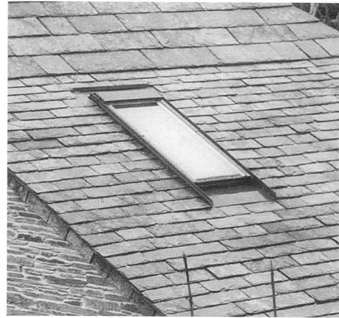
Rooflight of vertical format, neatly set into the roof.
