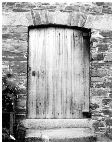
An unstained oak boarded door weathers to a silver grey. This would be suitable for a rural property.
