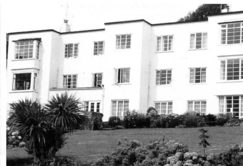
When replacing windows match the glazing pattern to suit the period of the property. Horizontal glazing patterns are typical of the interwar period.
