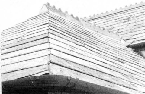
Scalloped terracotta ridge tiles are a feature of the district. Note also the mitred hip.
