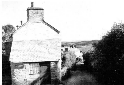
Chimneys are an important feature of a roofscape, adding interest and accent.
