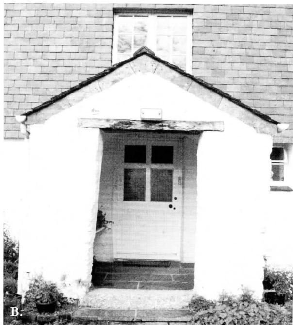
B. Traditional cottage porch. Note the slate verge and timber lintel. This one has a pair of benches inside.
