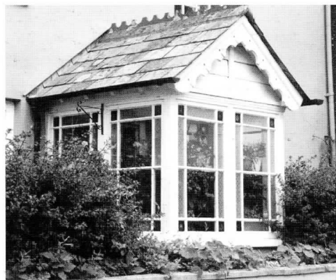
A small Victorian semi glazed porch. Avoid very ornate decorated timber work, unless faithfully reproducing high 'Victorian' detailing on a property of that period.
