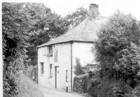
Painted stonework and slate roofs are typical of many rural villages.
