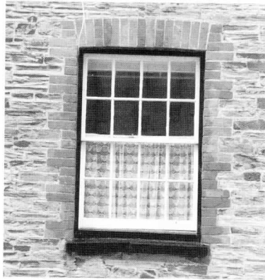
The window above has a segmental arch with brick quoins.
