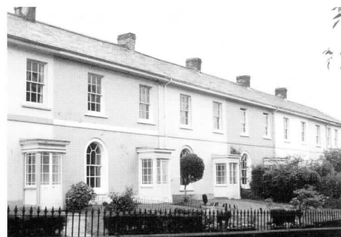
Smooth pastel coloured painted stucco lends this Georgian terrace a refined character. This finish is most suitable for formal style buildings.
