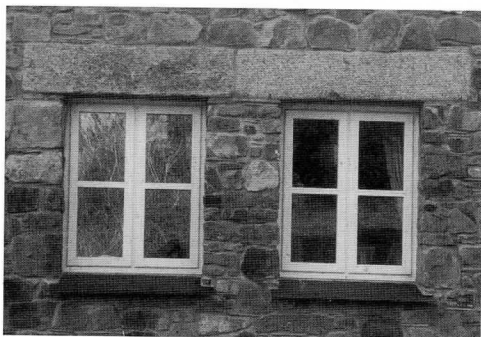
Massive granite lintels are a feature of the Cornish vernacular.
