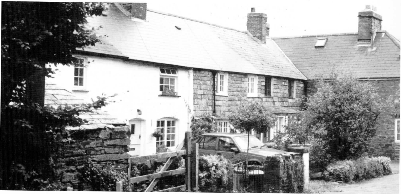
A charming group of cottages near Tideford. Frontages are a mixture of slate hanging and white painted stone work.
