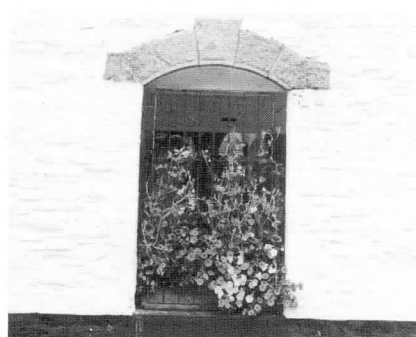
Granite arched lintels and brick Jambes are an unusual combination on this harbour front building in Looe.
