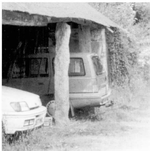
A traditional linbaw with granite post supporting the roof timbers.
