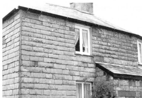
Slate hanging using large wide slates.
