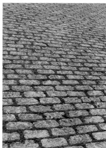
Tumbled concrete setts (grey) make a good modern alternative to granite. Avoid herringbone laying patterns.
