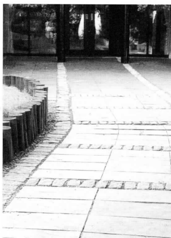
Riven slate and granite setts are a good combination of typically Cornish materials.
