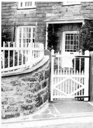
These traditionally detailed white timber painted fence and gate provide an appropriate boundary treatment to a Georgian country house.
