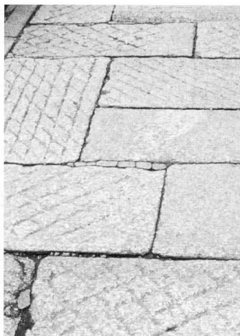
Large granite slab paving in Liskeard.
