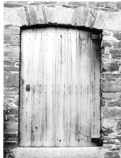
This modern oak boarded door is simple, robust, and weathers to a silver grey which tones in well with the local stone.
