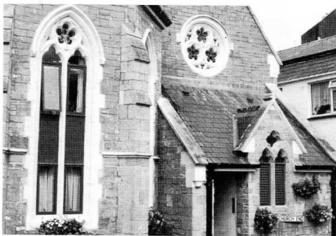
Church conversion at Looe which retains the wealth of original features, but the use of powder coated metal windows provides a more contemporary feel.
