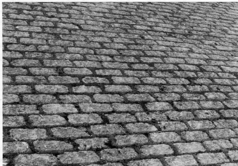
Tumbled concrete blocks.
