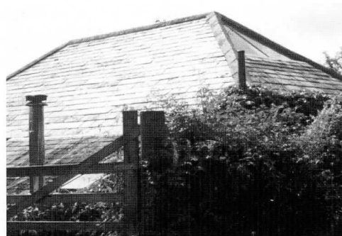
Barn conversion near Lostwithiel. Note the stainless steel flue and the unusual sky light - both features are appropriate to a conversion.
