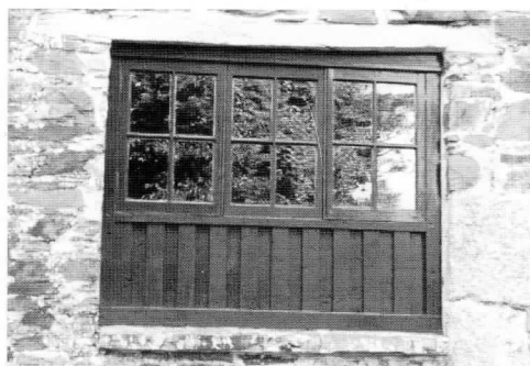
Note the infill panel under the windows, reminiscent of the slatted vents often found in stables or sheds. Subtly but significantly different to tongue and grooved boarding, which is to be generally avoided.
