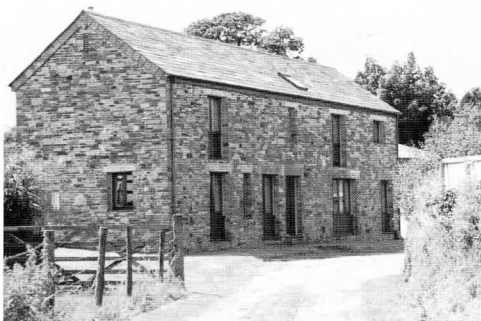
Barn conversion, East Taphouse. Note the deep reveals to the door and window openings. The use of traditional barn door and window vent joinery, and the use of dark stain rather than mahogany colour would have been more appropriate.
