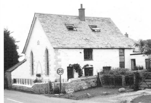
Chapel conversion at Minions which retains the charm of the original building, but has lost some of the ecclesiastical character by the addition of casement windows and chimney.
