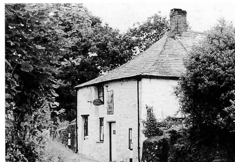
Mitred hips, slate roofs with terracotta ridges and chimney are traditional details in the district.
