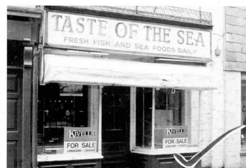
A characterful old shop front at Liskeard. note the panels on the stall riser.
