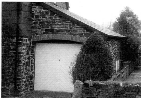
A well designed garage with associated stone walls and planting; it could be improved by the use of a vertically boarded door, rather than the chevron pattern.
