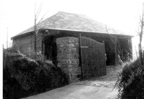
A car port based on a traditional lincay or cartsbed, is very suitable for rural areas. Note the use of natural slate and stone in this example.
