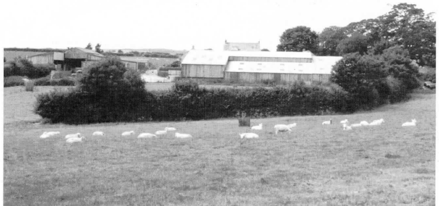
The 'breaking up' of planes of roof help to reduce the apparent bulk of this barn in the surrounding landscape.
