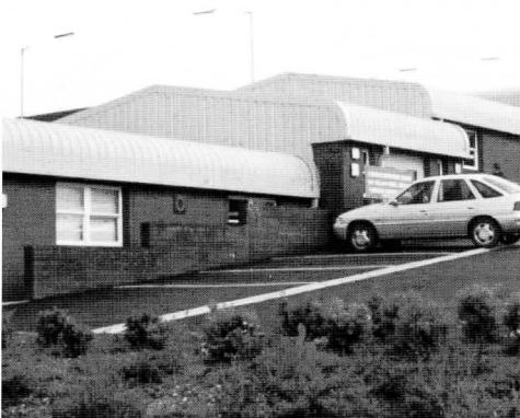
An interesting roofscape can help reduce the apparent mass of a building.
