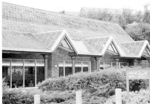
Foreground planting helps to 'anchor' buildings.
