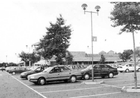
Tree planting and lighting play an important part in softening the effect of large car parking areas.
