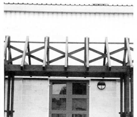
Pale cladding colours are helpful in blending a building into the sky.
