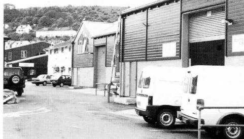
The fish market at Looe. A series of simple large sheds using contemporary materials, but through sensitive handling of scale, materials and colour retains a strong local identity.
