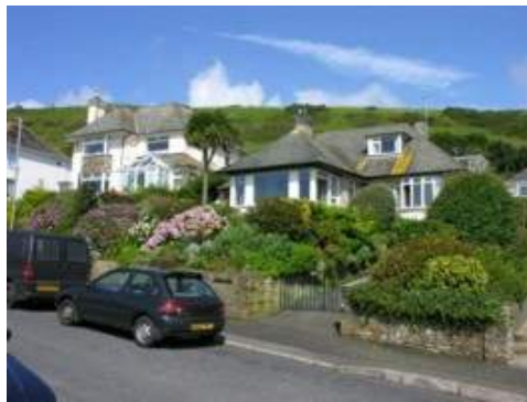
79: A quite standard bungalow enhanced by its random slate roof with mitred hips
