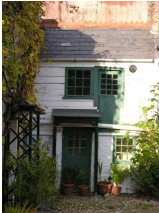
70: A great example of a small scale working yard and buildings
