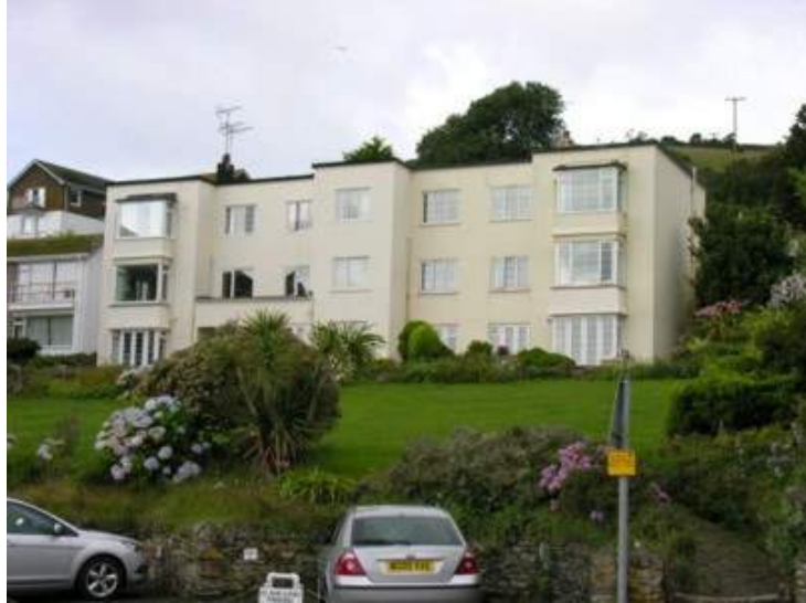
17: Loss of character affects buildings of all ages
