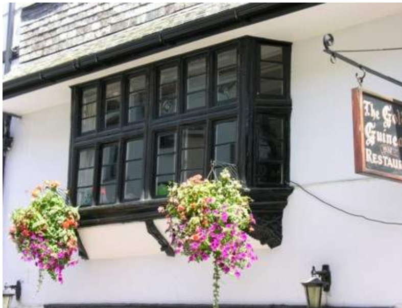
8: A 17 th century oriel window with decorative brackets. It would have had leaded casements originally.
