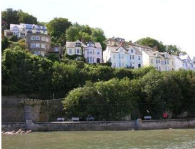
77: Architecture and engineering at Hannafore Road
