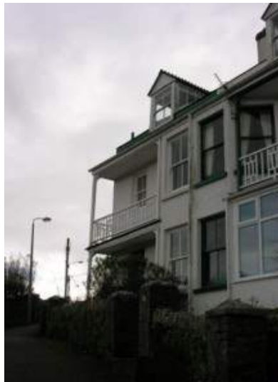
67: Good detailing at Furzedown Terrace
