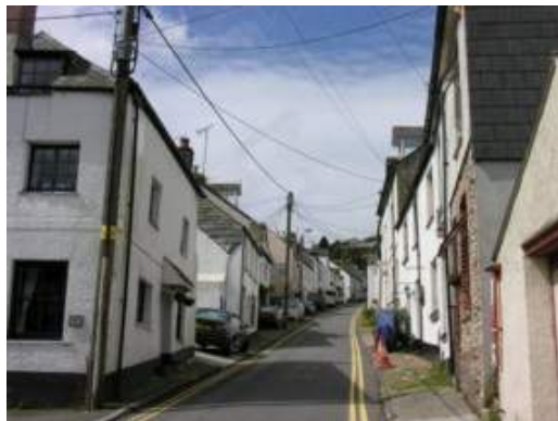
37: Intrusive wirescape in West Looe
