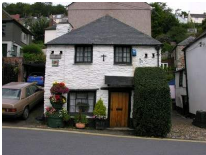
18: Painted rubble stone on an historic cottage
