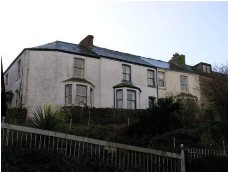
65: Survival of original windows at Beech Terrace
