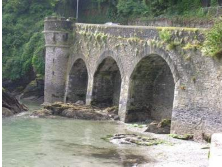
13: The picturesque engineering solution at Hannafore Road
