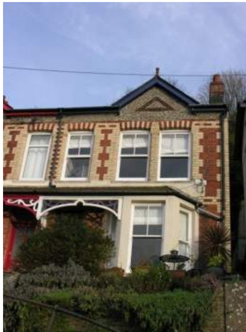
14: Attractive details on a late Victorian terrace
