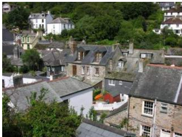
22: The topography means the roofscape is key
