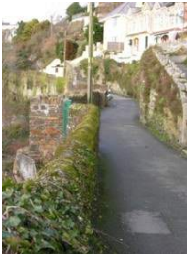
55: Massive retaining walls mark the historic link between Shutta and East Looe
