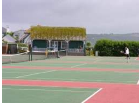
78: The tennis pavilion is a focal point
